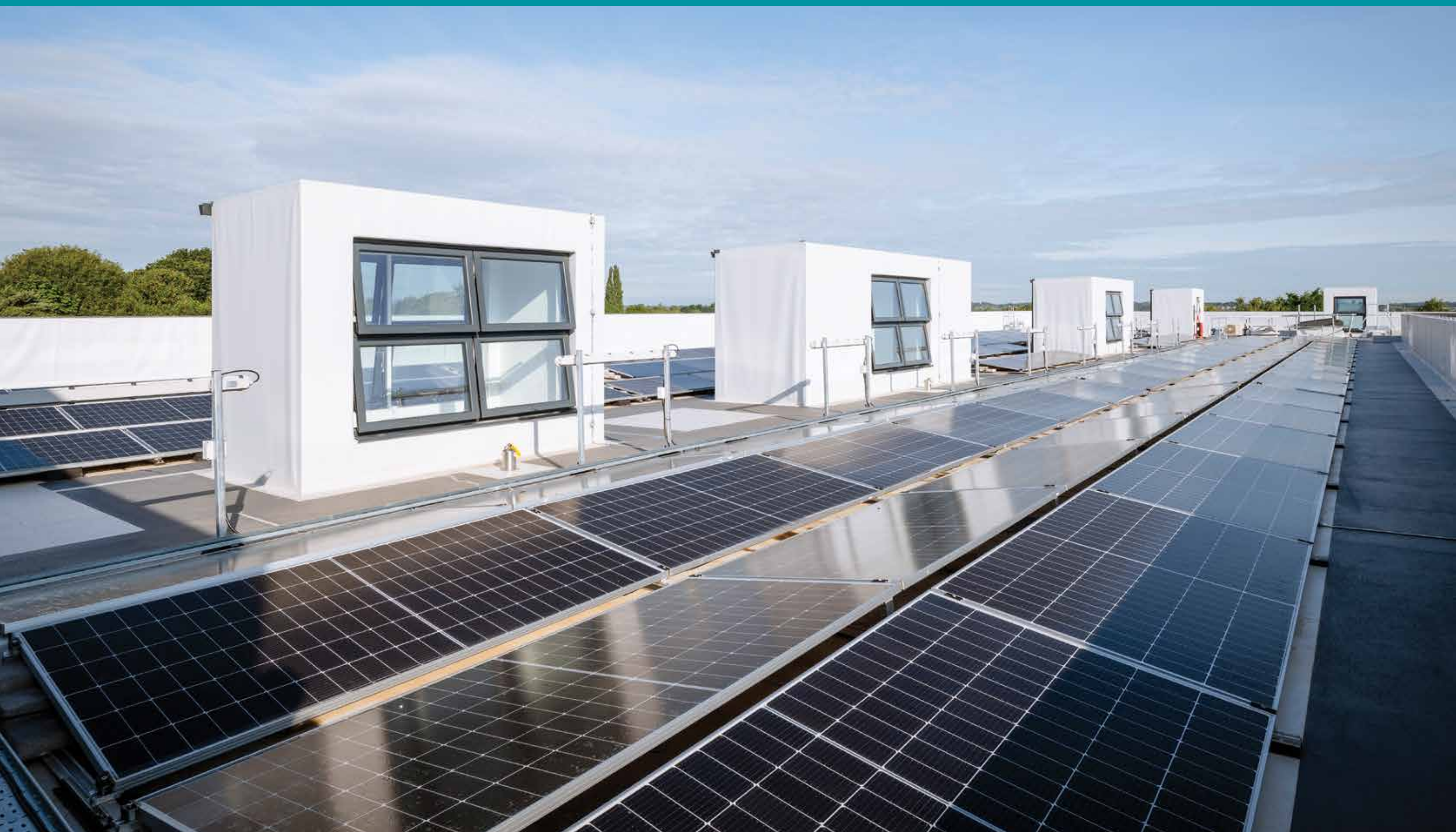
Photo showing PV panels installed by Bowmer + Kirkland at Belvidere School, Shrewsbury.
